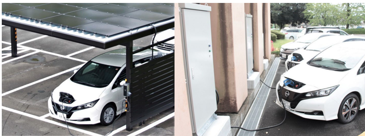
Figure 5-6 Ongoing demonstration at Kunitomi-cho of an energy management system that uses solar power, battery storage, and EVs 27
